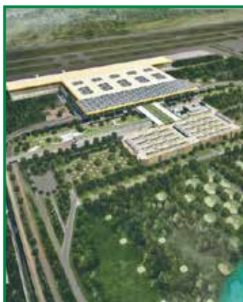
New Yogyakarta Airport Yogyakarta, Indonesia
